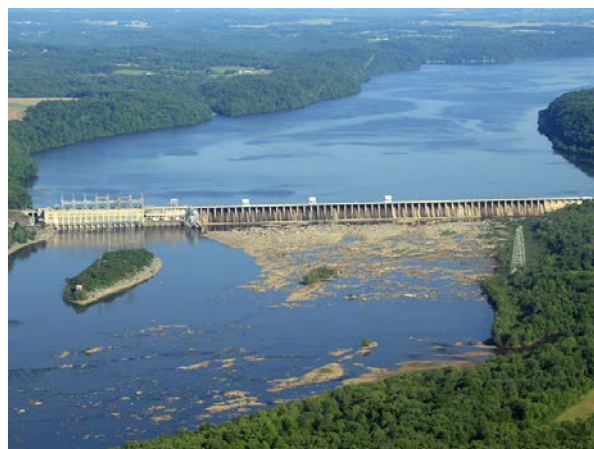
Conowingo Dam is a large hydro-electric dam near the mouth of the Susquehanna River. (Photo: Jane Thomas, Integration and Application Network, University of Maryland Center for Environmental Science)
